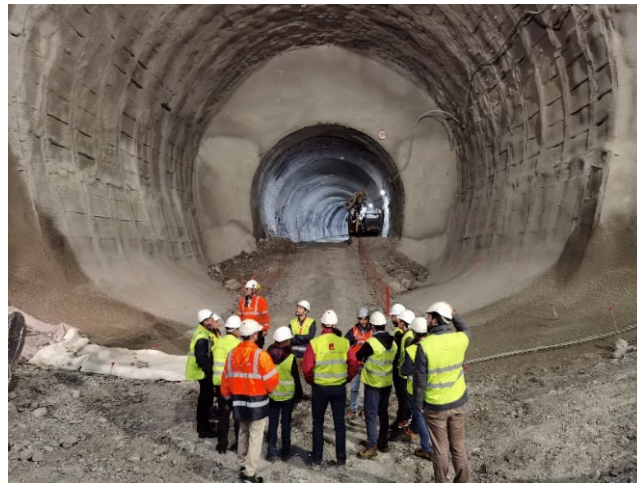
Fig.8. Image of the excavation of the Lisbon metro lines.
